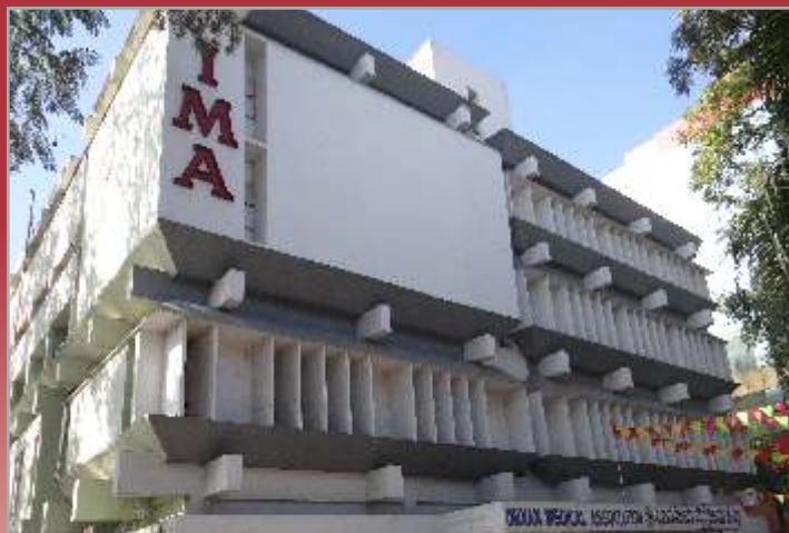
IMA KSB Building
